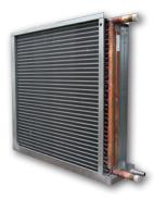
Water is cooled in the cooling unit. Cold water is pumped into a cold water battery in the air handling unit. This will cool the air flow.
